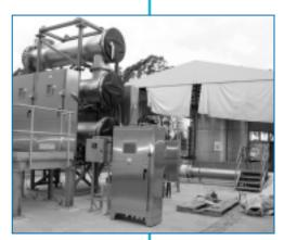
Construction of the Phox advanced oxidation ultraviolet (UV) system by Trojan Technologies began in summer 2003. The GWR System will contain nine UV Phox systems, and each system will treat up to 8.75 million gallons of wastewater per day. When complete, it will be the largest UV treatment system designed for NDMA removal in the world.
